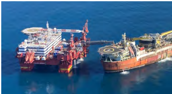
Floatel Superior at Balder FPSO for Vår Energi.
